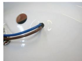
No grommet on the base of the fitting.
