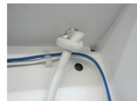
No gland used to secure cable to fitting.
